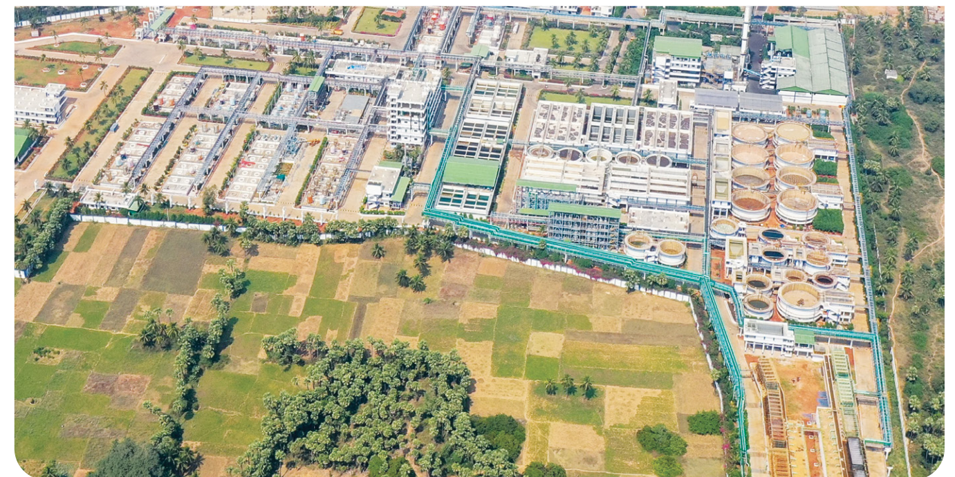
Unit 2 : Off-Ground Effluent Treatment Plant
