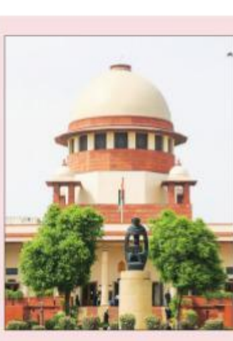
Supreme Court building in Chandigarh.
