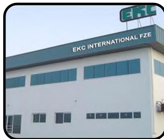
Plant II – Dubai
