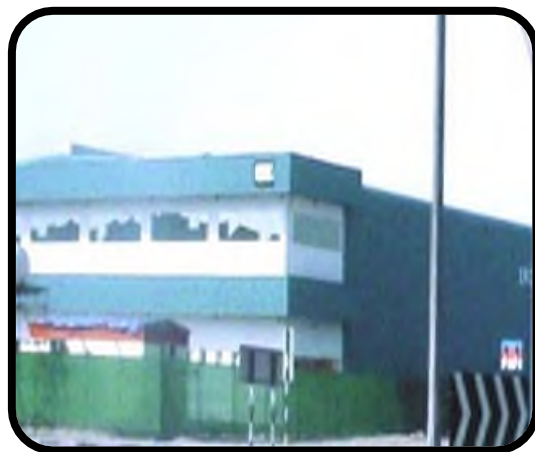
Plant I – Dubai
