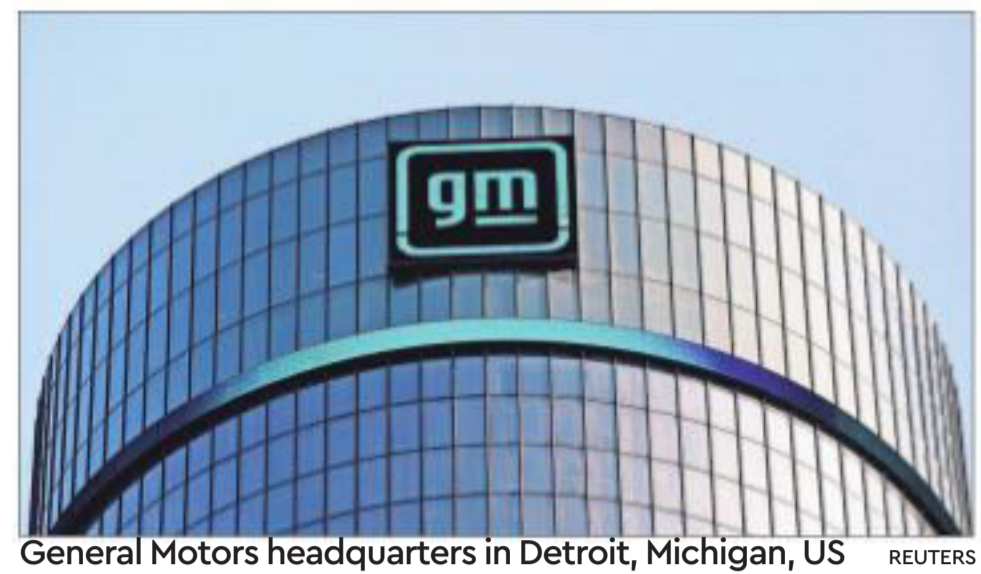
General Motors headquarters in Detroit, Michigan, US
