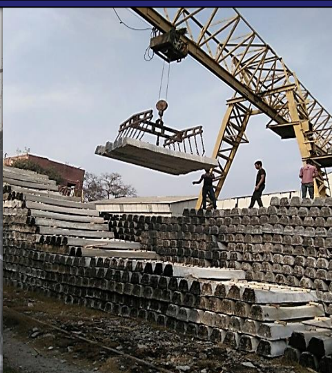
Sleeper Lifting work
