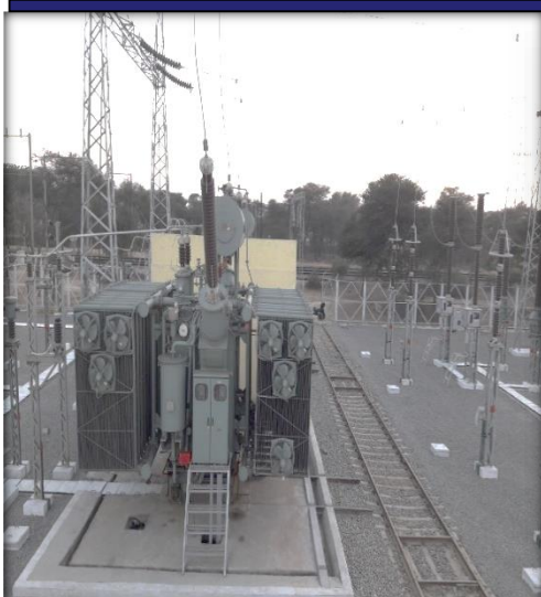
Traction Substation work
