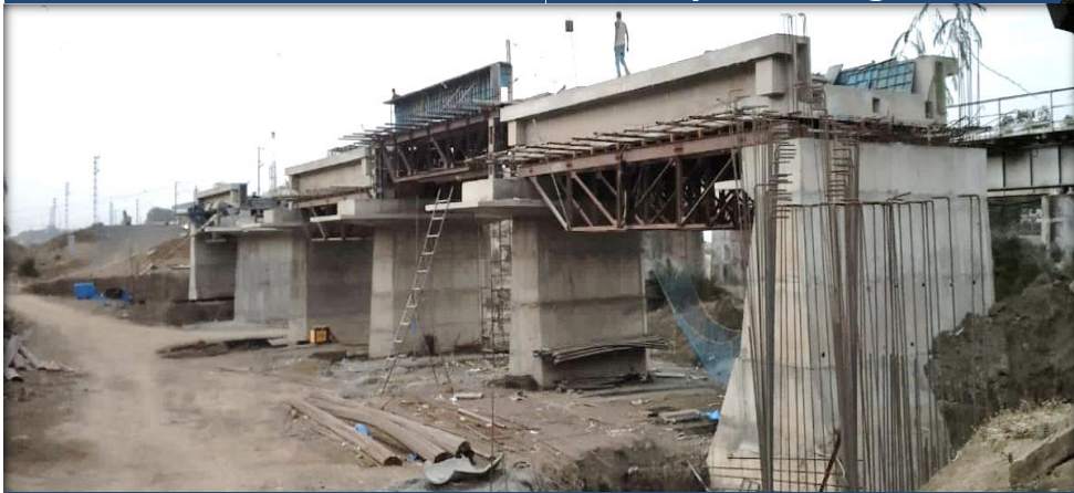
Major Bridge work at a Composite project
