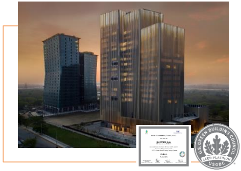
Max Towers - Certified LEED Platinum from USGBC and Health and Wellbeing Gold from IGBC
