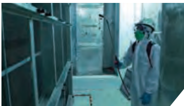
Enhanced AHU Cleaning
