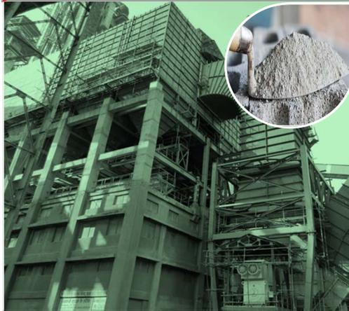
Thermax upgraded existing bag filter to RABH with 6 units of modules, addition to existing 10 units for a cement major in India.
