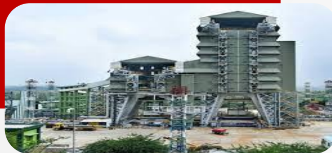
Received order for 86KL LH 2 Tank from India's space agency for their facility
