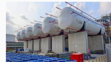
Hydrogen tank installation
