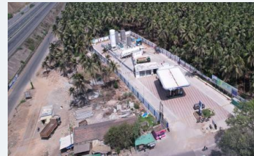
LNG/LCNG fuel stations
