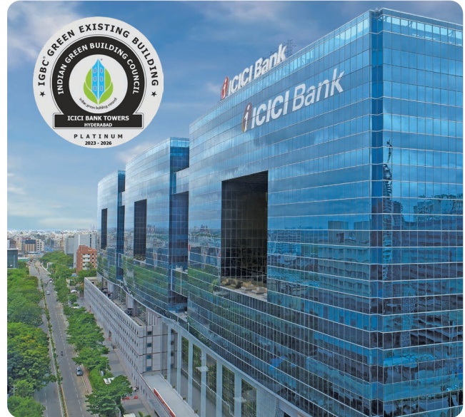
ICICI Bank office at Gachibowli, Hyderabad, rated 'Platinum' by IGBC in 'Green Existing Building' category (inset: IGBC Plaque).
