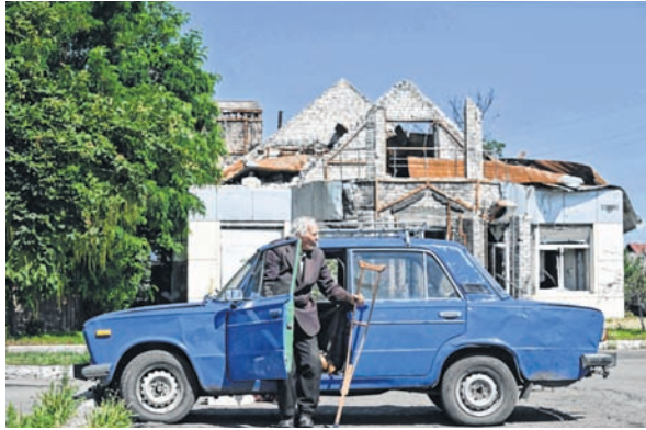
An elderly man exits a car in front of a heavily damaged building in Lyman, Donetsk region, on Monday
