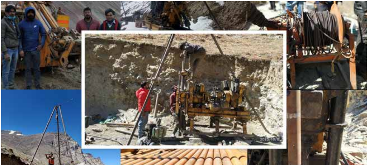
RITES' team undertakes geotech investigation for a tunnel project in Leh
