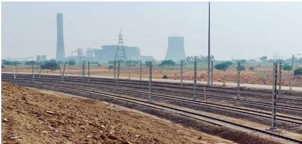
Project Management Consultancy for rail infrastructure at the Ghatampur Thermal Power Plant, UP
