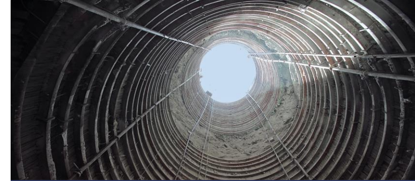
Rampur HE Project - Himachal Pradesh (432 Mw) Asia's largest Surge Shaft with 38m dia.
