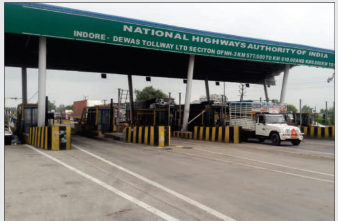
Indore Dewas Tollways Limited
