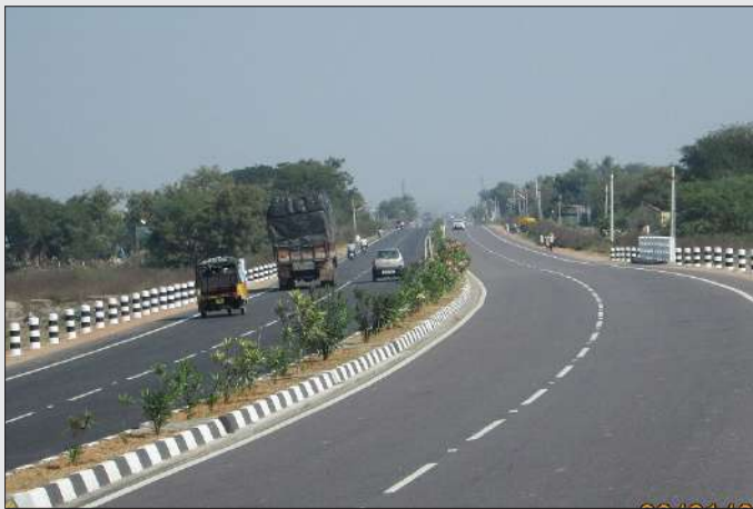
HKR Roadways Limited
