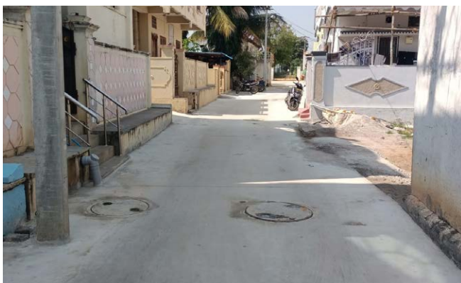
Underground Drainage and other rural development projects in Tangatoor, Shankarpalli near Hyderabad.
