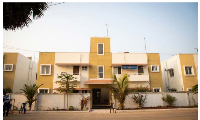
Construction of Rural Housing and Other Rural Development Projects in Antervedipalem, EGDT, A.P.
