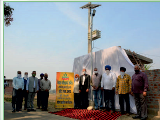
NFL installed 325 Nos. Solar Street Lights in nearby villages in Nangal, Punjab
