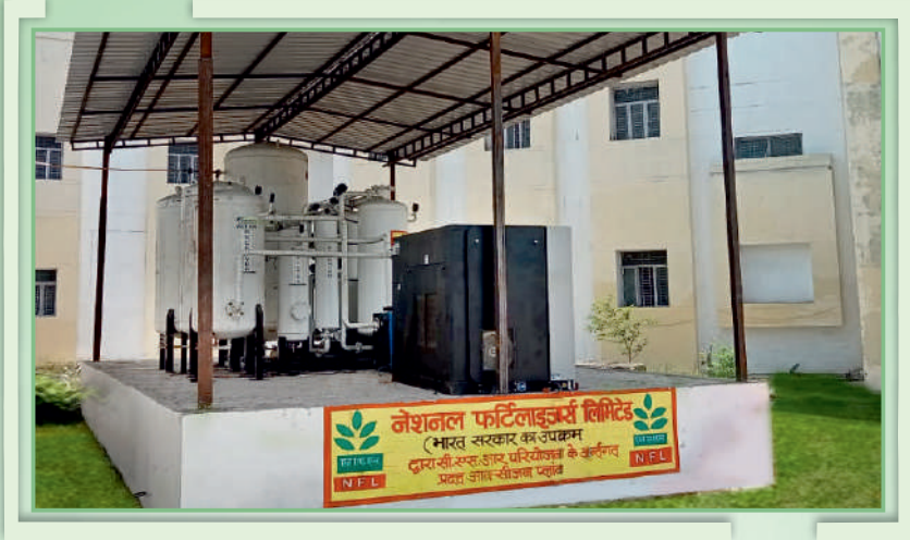
The company installed & commissioned 04 nos. Medical Oxygen Generator Plants at Bhopal, Lucknow, Gorakhpur & Indore to strengthen the Covid Care facilities
