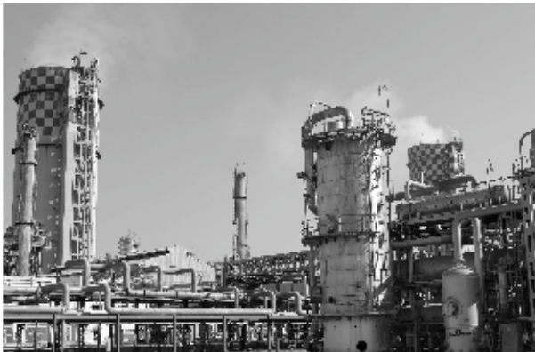
VIJAIPUR I & II PLANT
