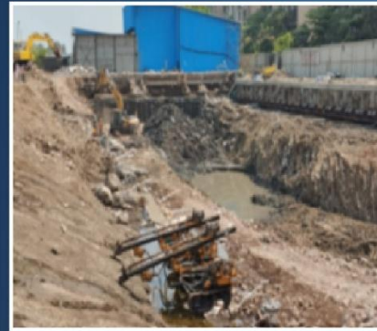
Piling Work Completed May 2022
