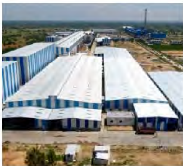
TNPL's Board Plant - Unit II
