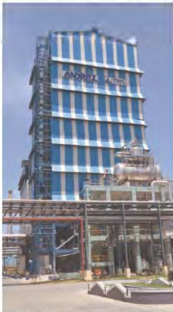
View of the Chemical Recovery Boiler in Unit - II
