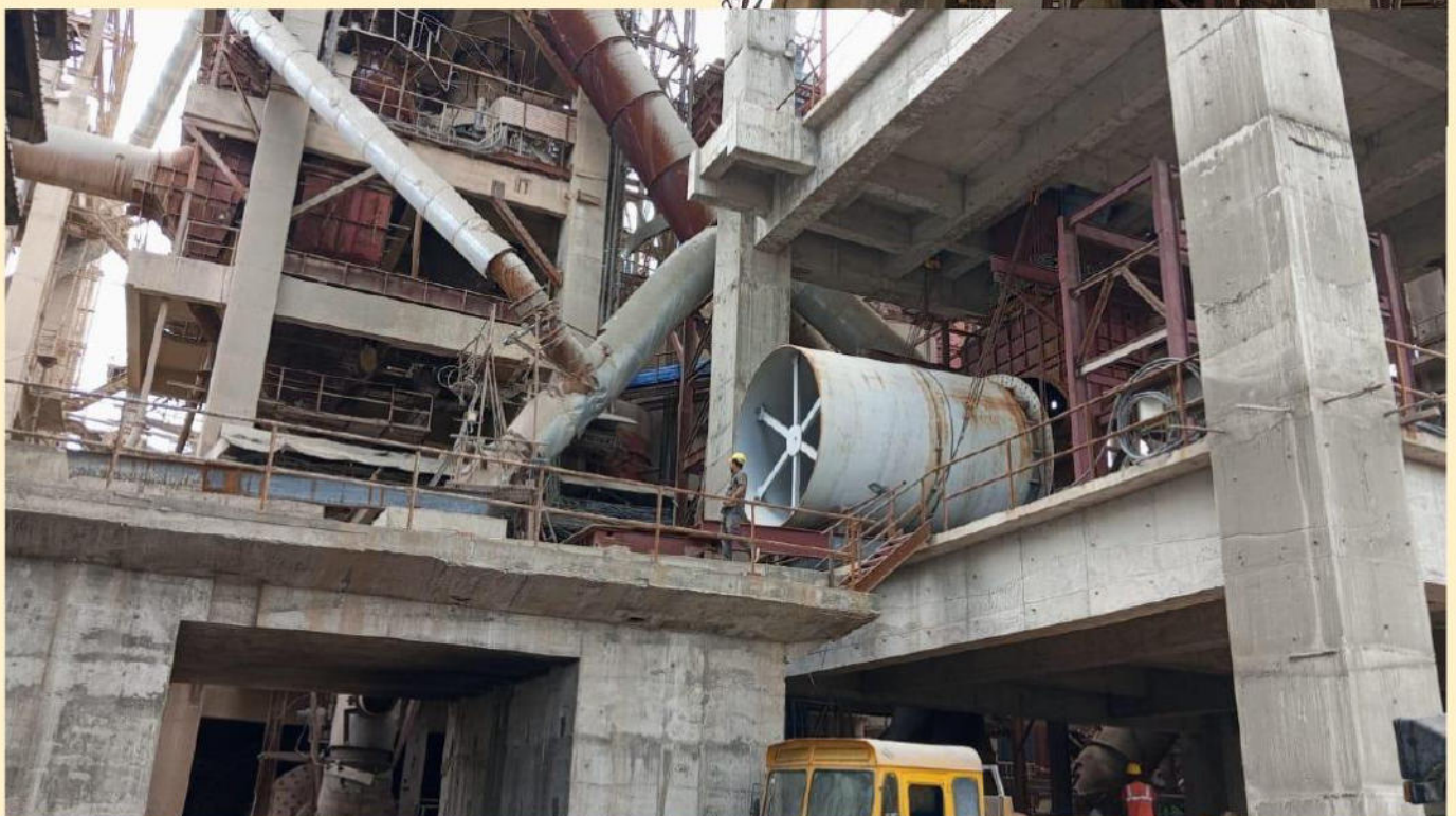
Kiln installation in progress.....
