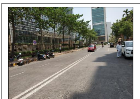
View of Access Road
