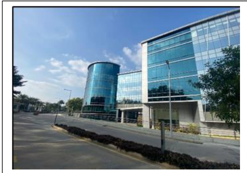
External view of the subject property (SP)
