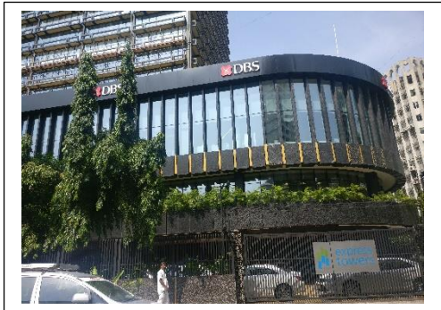
External view of the subject property (SP)
