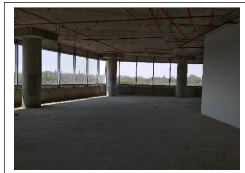
Internal View of office area
