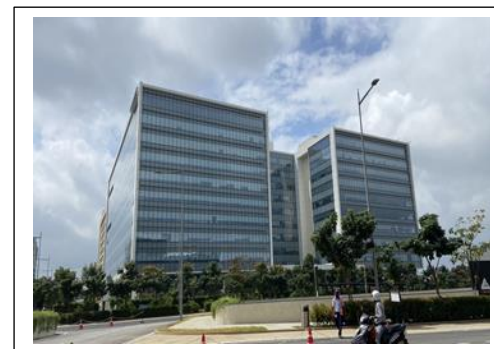
External view of the subject property (SP)
