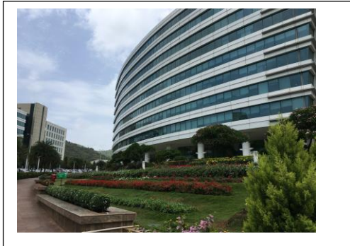
External view of the subject property (SP) ~ Block 4
