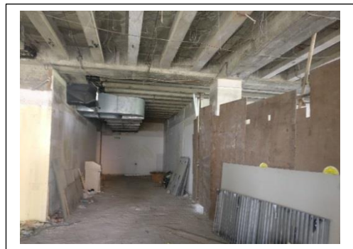
Internal view of a specific vacant unit in Subject Development
