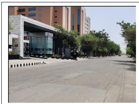
View of the primary access road/entrance
