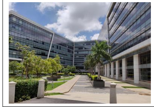
External view of the subject property (SP)
