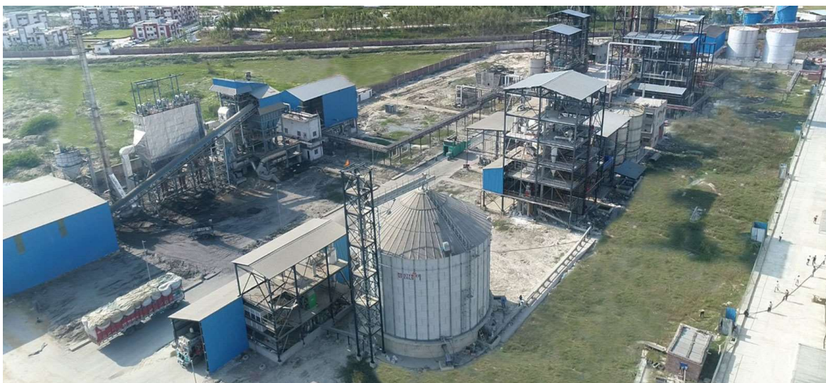
Sandila Plant, Dist Hardoi (U.P.)
