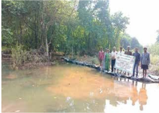
Check Dam: Moravane, Chiplun, Ratnagiri
