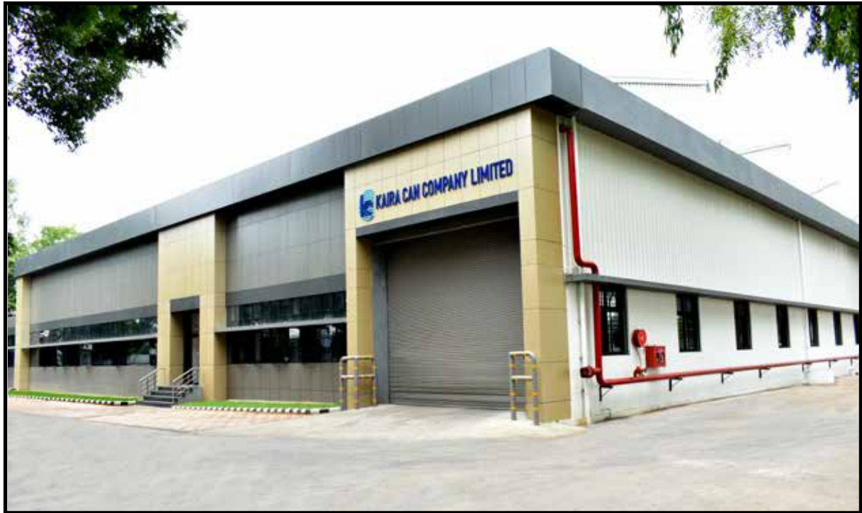
Kanjari Factory - Gujarat
