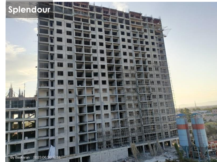
Project Status as on Jun 2023
