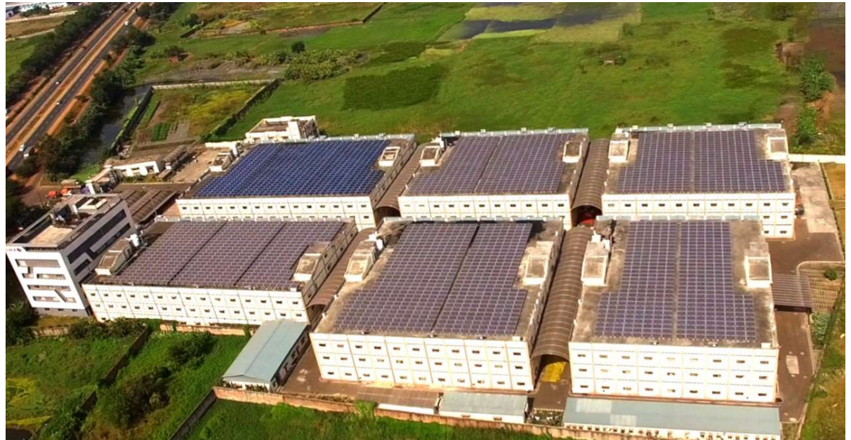
Rooftop solar power plant at Dankuni unit
