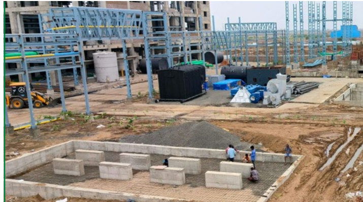
Foundation Works Completed of Isobutylene (RM) Tank
