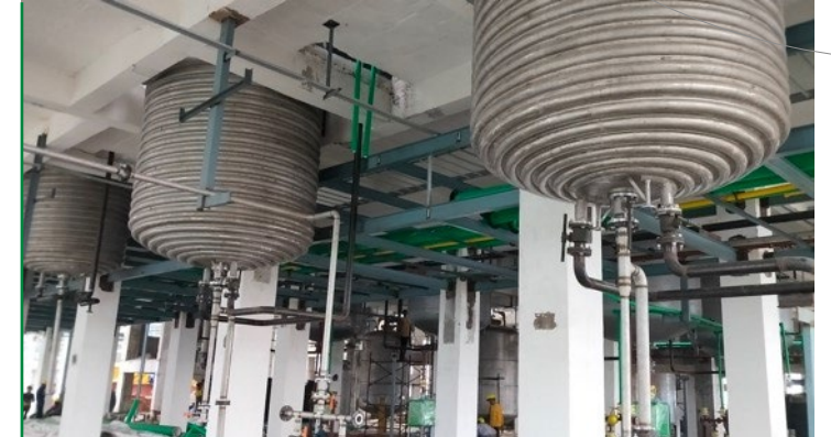
Reactor Installation
