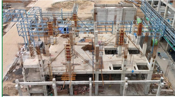
Civil Works at Recovery Plant
