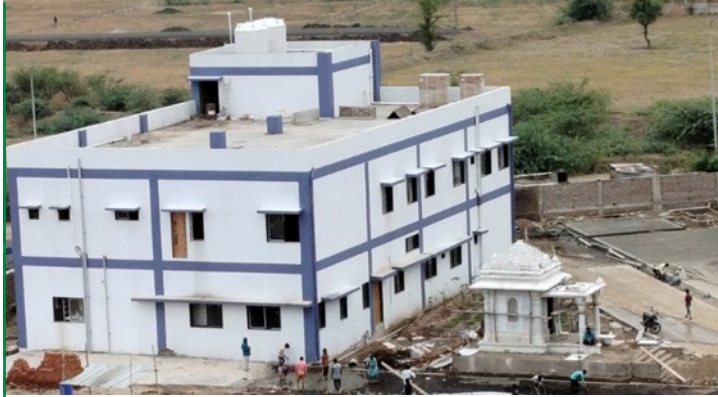
R&D and Administration Block Started in July
