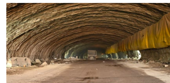
Vadodara-Mumbai Expressway, IRCON
