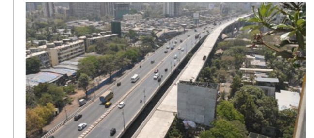
Santa Cruz-Chembur Link Road Flyover
