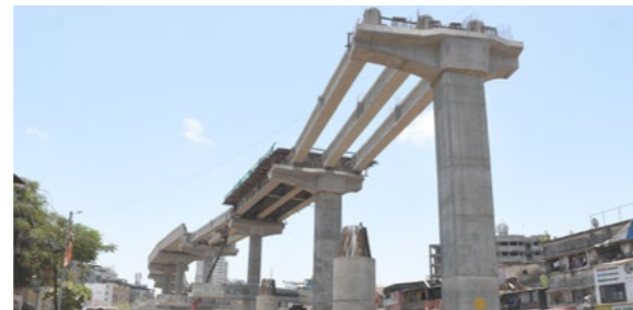
Mumbai Metro Line 9
