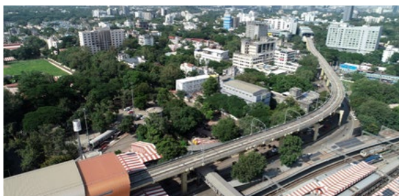
Pune Elevated Metro
