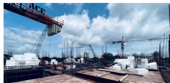
Pune Underground Metro
