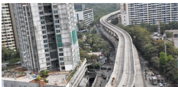
Mumbai Metro Line 6
