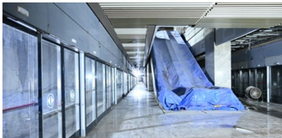
Mumbai Underground Metro Line 3
