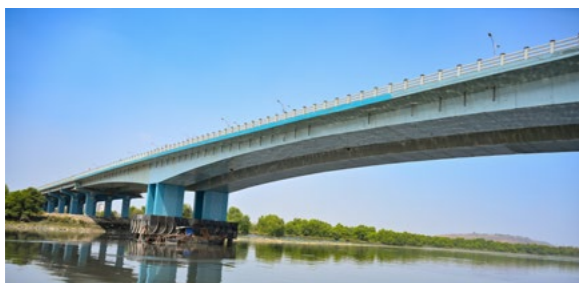
Motagaon Creek Bridge
