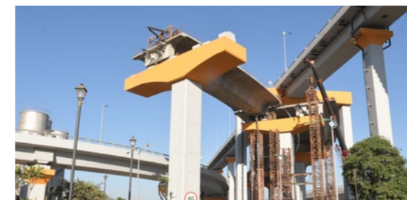
Sewri-Worli Elevated Flyover
