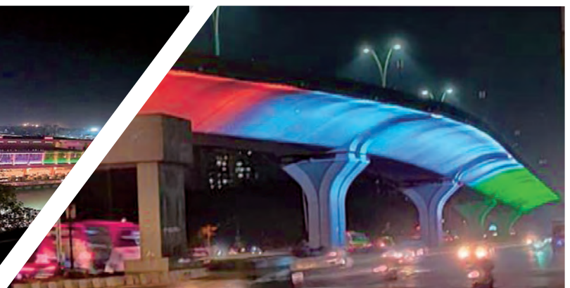
BKC Connector Bridge, Mumbai
