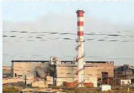
CAPTIVE POWER PLANT
