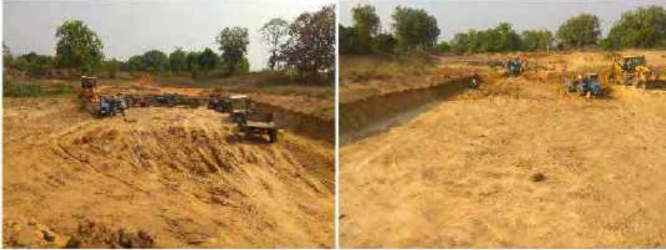
Water Pond excavation in Navapara village under CSR Activity
