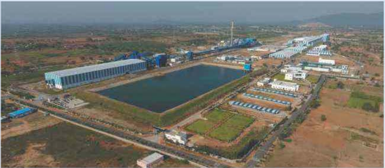
Bird's eye view of TNPL Unit II – As seen from Eastern side
