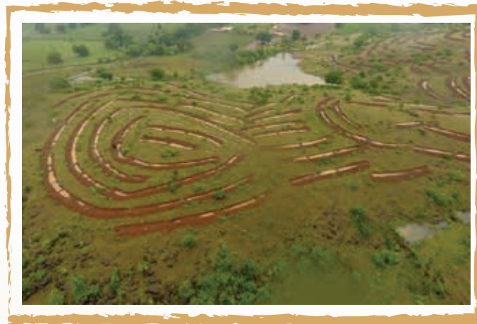
Deep Continuous Contour Trenches
