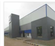
Foundry Division, Vambori
