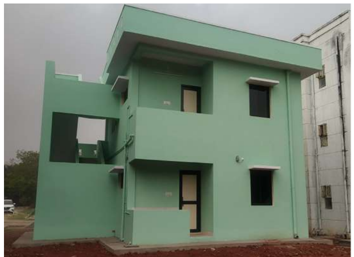
NACA Building at Simhadri
