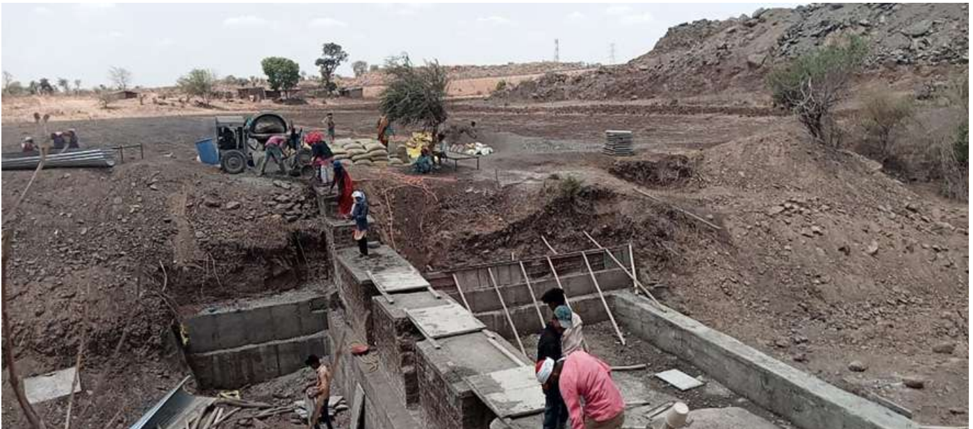
Ongoing Stop Dam Renovation Work at Village Aarsi Under NLRP
