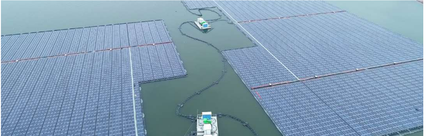
NTPC Ramagundam Floating Solar
