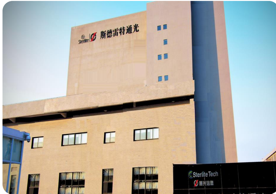
Optical Fibre Facility, China
