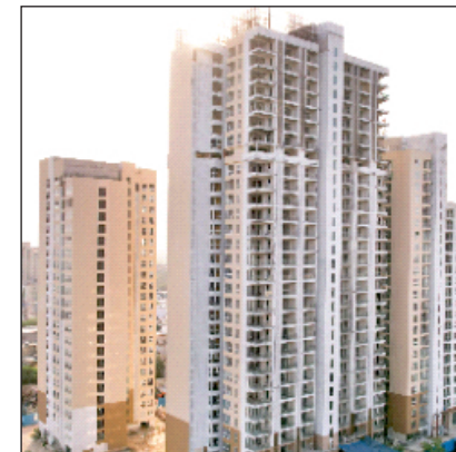
Godrej South Estate, NCR 0.58 million sq. ft. GPL Economic Interest : 100% owned project
