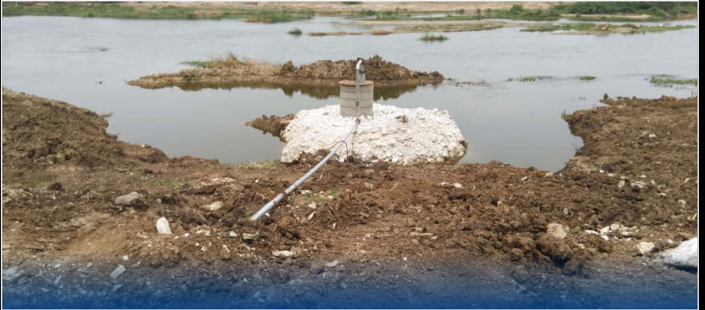
Filter bed arrangement at TRCL Jayanthipuram Plant Mines for providing irrigation facilities to nearby villages
