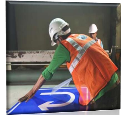
ROAD SIGNAGES AND MARKING PAINT
