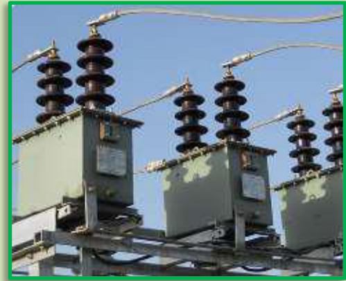
MV Current and Voltage Transformer upto 33 kV
