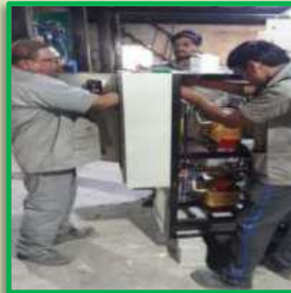
Busbars worksControl wiring
