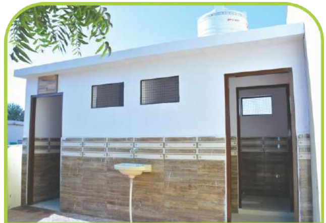
Constructed New Toilet for Girls & Boys in various Govt. School in nearby Jaipur
