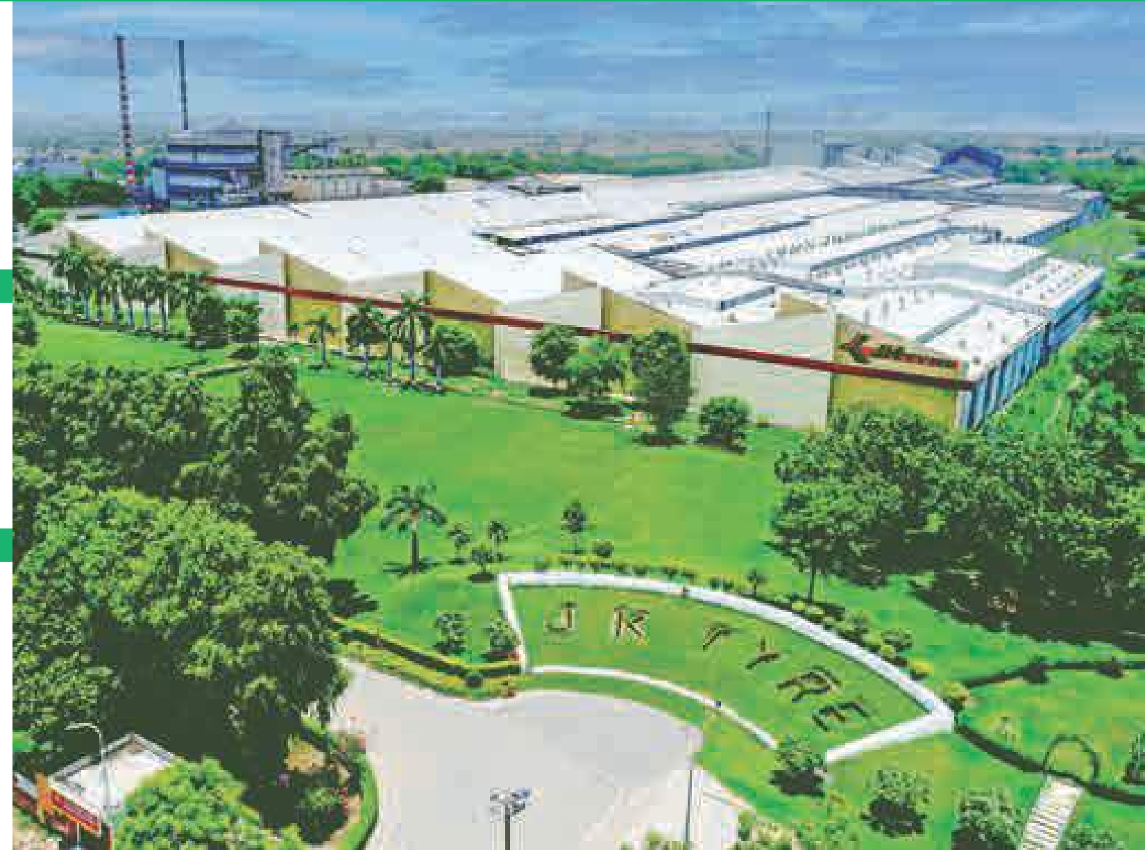
JK Tyre Plant, Banmore, Gwalior
