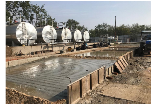
Surface Facility augmentation at Karjisan
