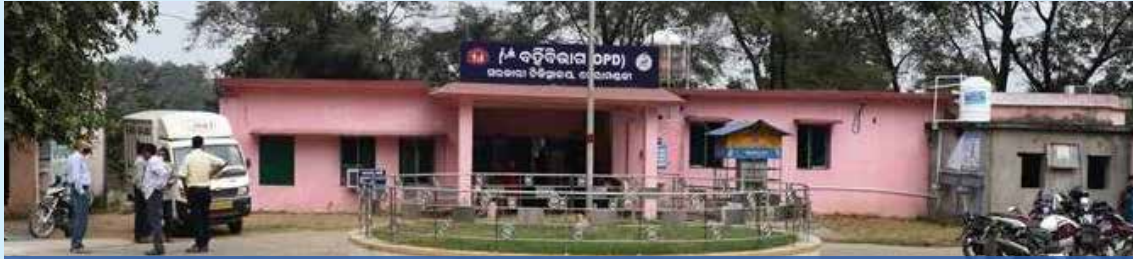
Before Renovation of Primary Health Centre
