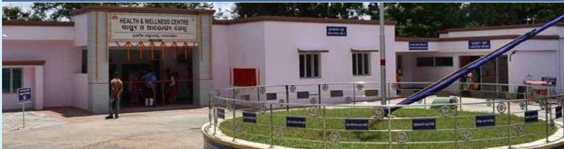
Renovated Primary Health Centre
