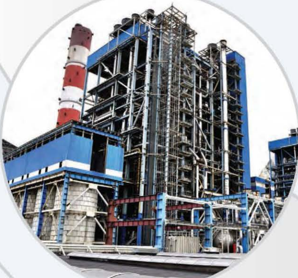
660 MW Super Critical Steam Generator - NTPC Solapur Thermal Power Plant
