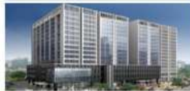
HQ and R&D center
