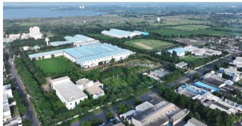
Manufacturing Facility, Rajkot
