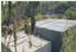
Positioning and constructing new site establishments carefully between existing trees to protect them
