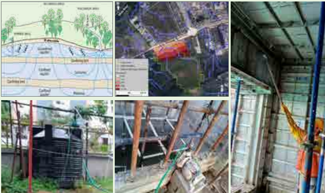
Use of curing compound instead of water Rainwater storage and reuse for curing
