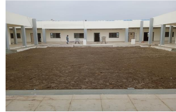
Construction of ITI at Panna
