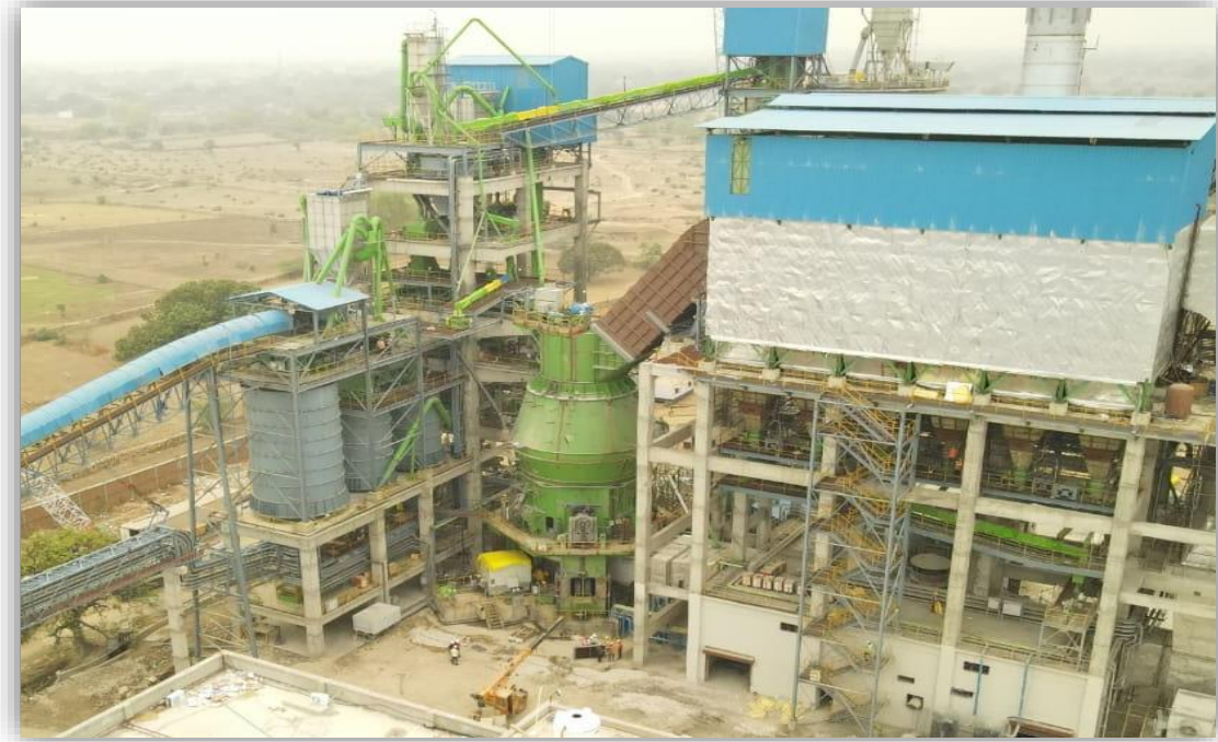
Hopper & Cement Mill
