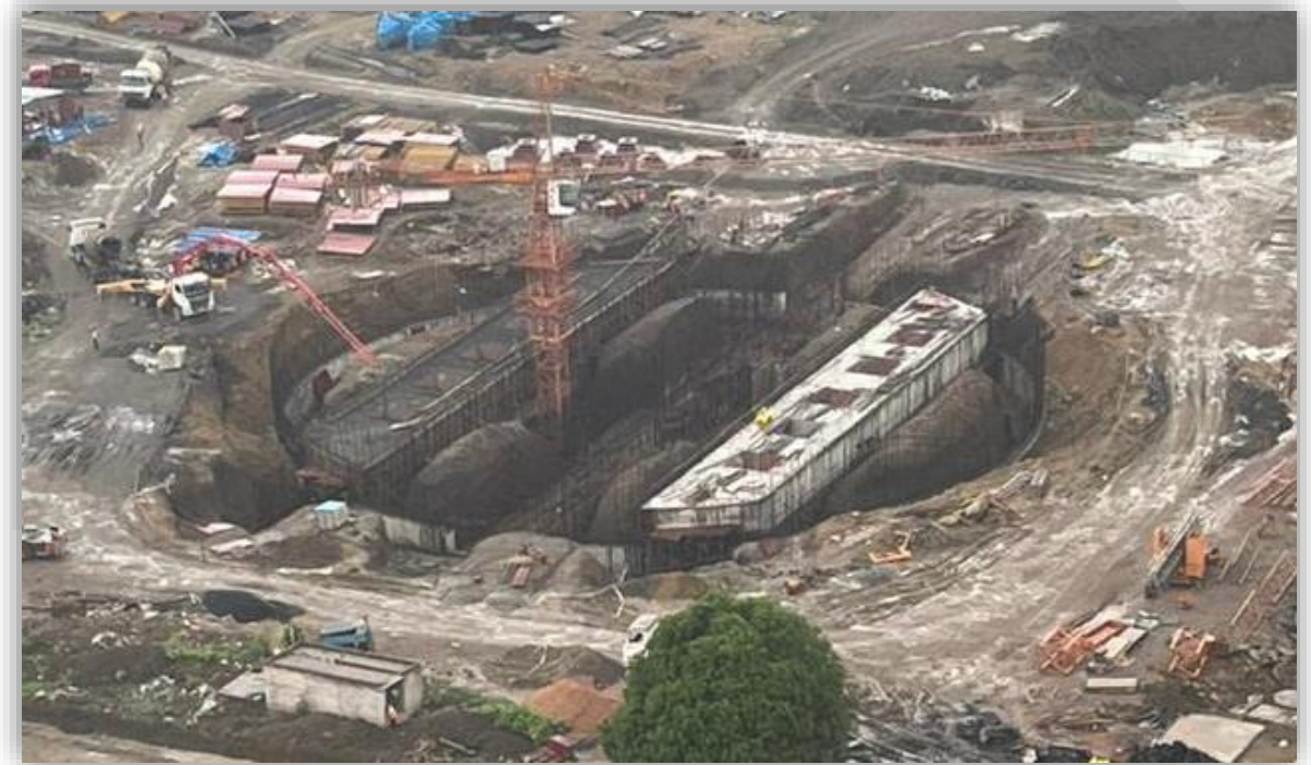
Clinker Silo Slab Casting
