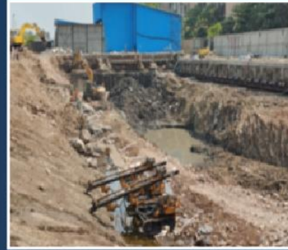
Piling Work Completed May 2022
