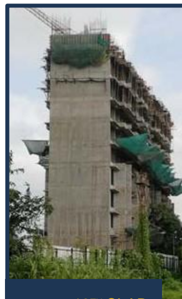
( SEP-21 ) 13 TH SLAB
