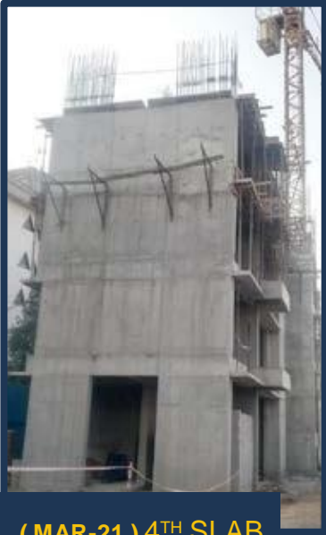
( MAR-21 ) 4 TH SLAB
