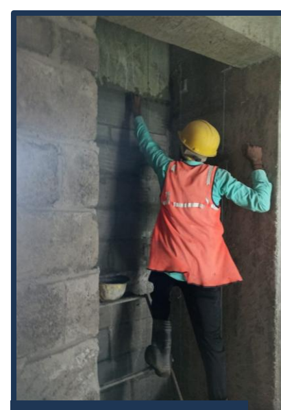
( JUL 22 ) INTERNAL PLASTER (WIP)
