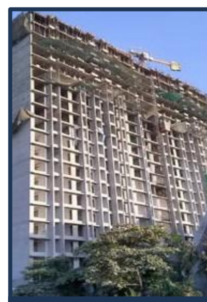
( FEB 22 ) SUPER STRUCTURE COMPLETED
