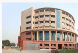
Supreme Court of India – Extension Building, Delhi
