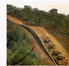
Panvel Dabhol Pipeline Project–Gail Ltd - Maharashtra
