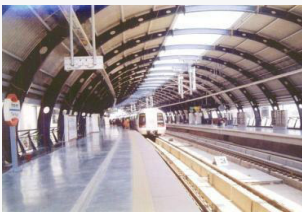
Elevated Metro Stations, DMRC, Delhi
