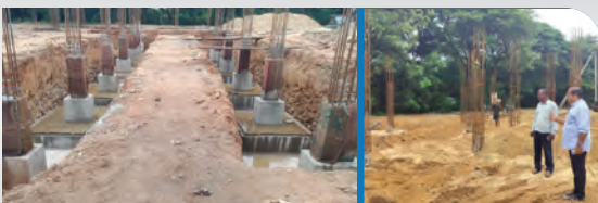
Contributed towards construction of Women's hostel.
