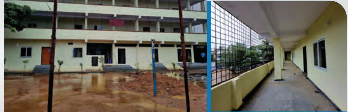
Contributed towards Construction of Zilla Parishad High School at Annaram Village of Sanga Reddy District of Telangana.
